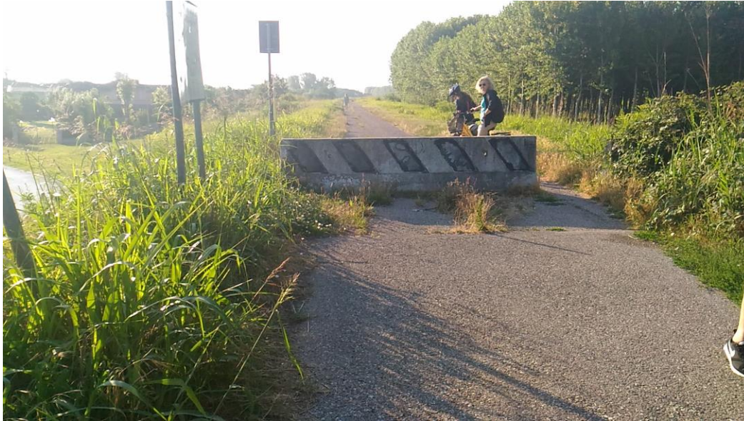
Chicane with less than 1.3 m clearance on daily section "81: Viadana (West border of Mantova Province on left riverside) - Borgo Virgilio" in Italy
